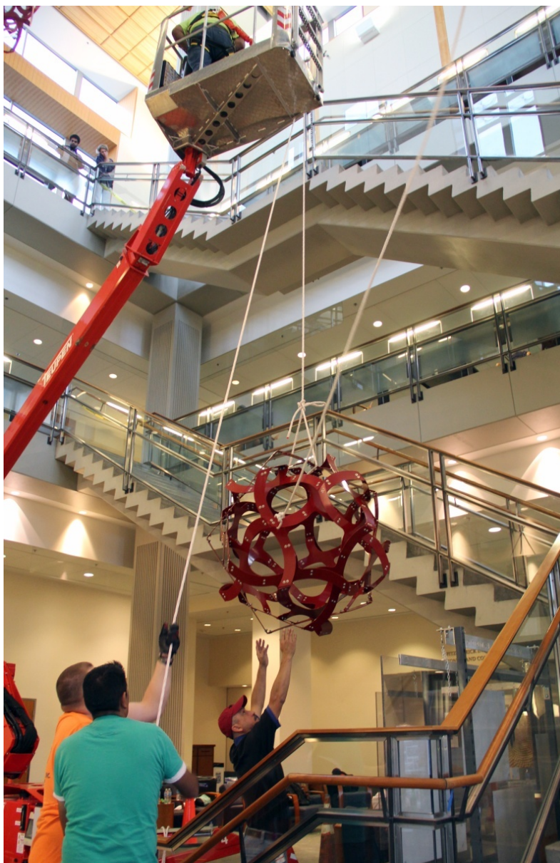
Figure 13: Riggers raise the orbs into position and attach them to the chains.
